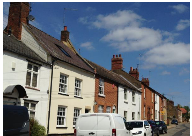
Terrace of cottages at Nos.22-28 High Street
