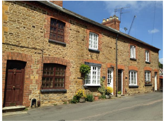
Stone and brick cottages at 2-8 Manor Road
