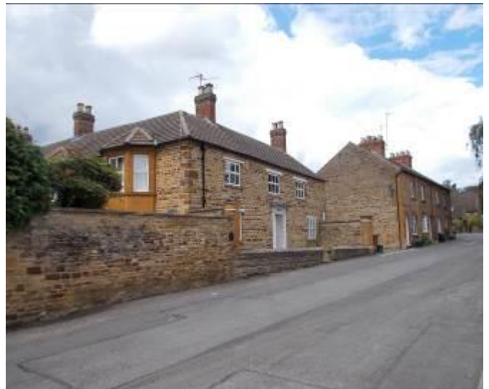
The Manor House and the cottages alongside form a significant group on Manor Road.
